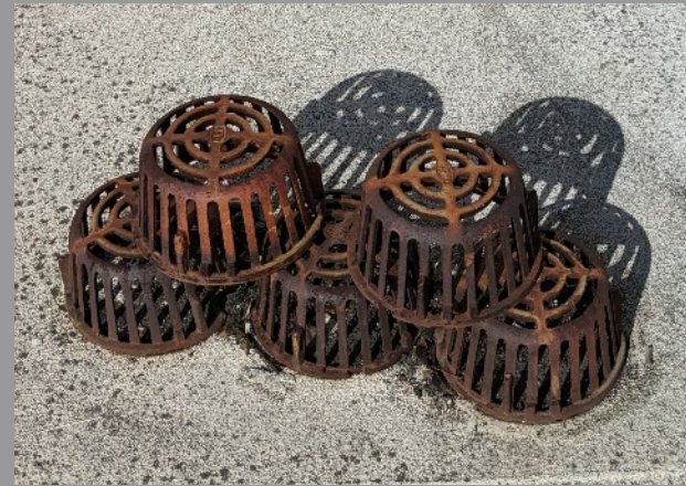
INSTALL (E) ROOF DRAIN DOME STRAINERS
