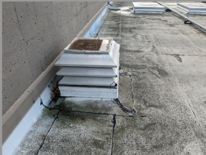
MISC. MINOR REPAIRS ROOF VENTS. REPLACE OR REPAIR TOPS.
