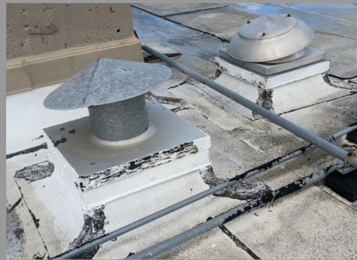
MISC. MINOR REPAIRS ROOF VENTS. REPLACE OR REPAIR TOPS.
