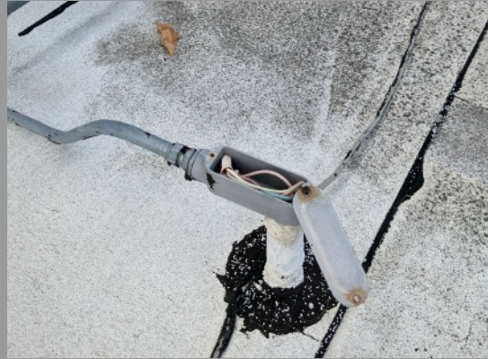
MISC. MINOR REPAIRS TO JUNCTION BOXES. FASTEN AND SEAL.
