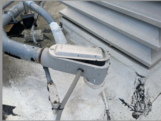
MISC. MINOR REPAIRS TO JUNCTION BOXES. FASTEN AND SEAL.
