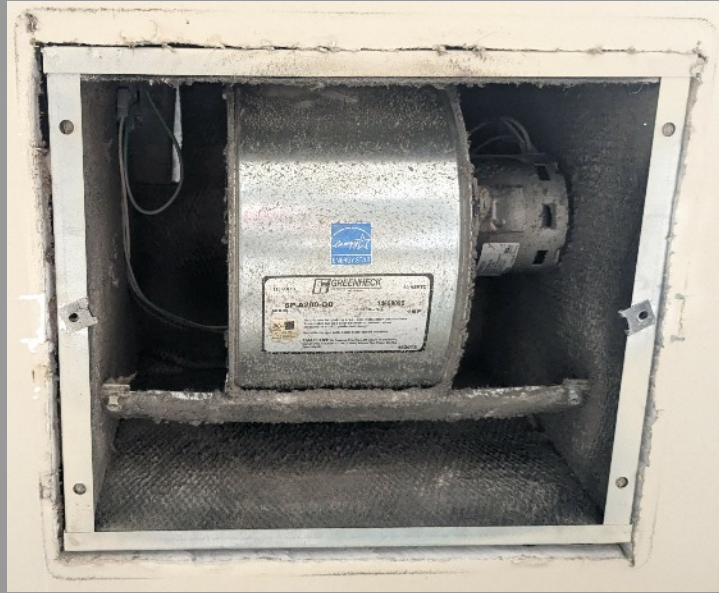
(3) LOCATIONS: 59, 79, 80 (E) MODEL GREENHECK SP-A200-QD
