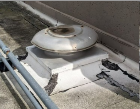
REPLACE VENT CAP NEAR ROOMS 61+62
