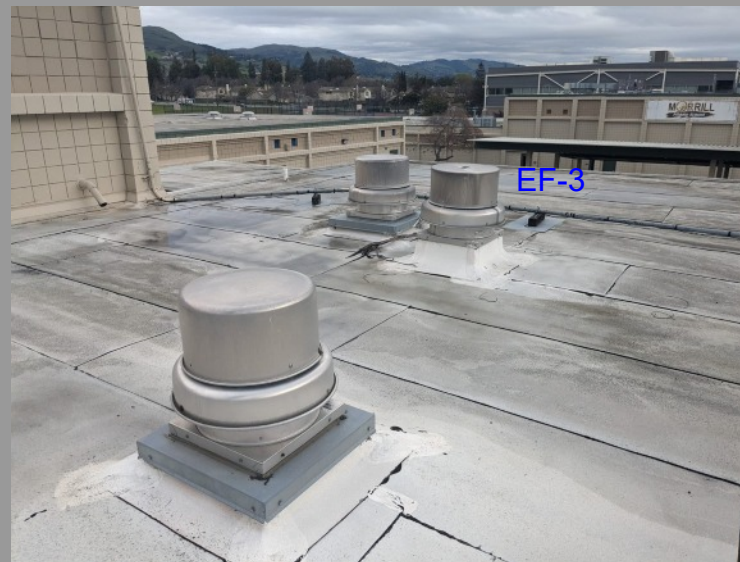
EXHAUST FANS SERVING THE RESTROOMS
